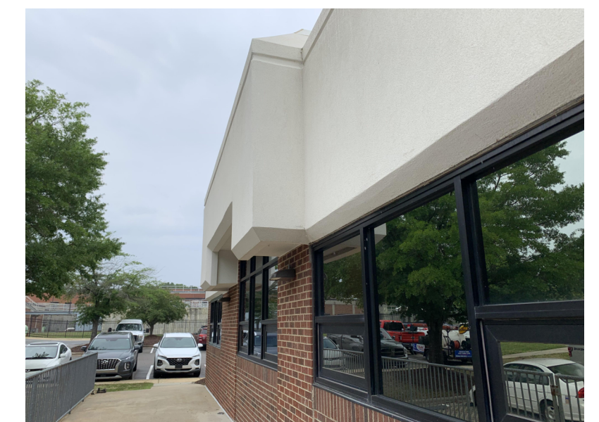
VIEW OF NORTH ELEVATION LOOKING EAST TOWARD WATER TREATMENT PLANT
