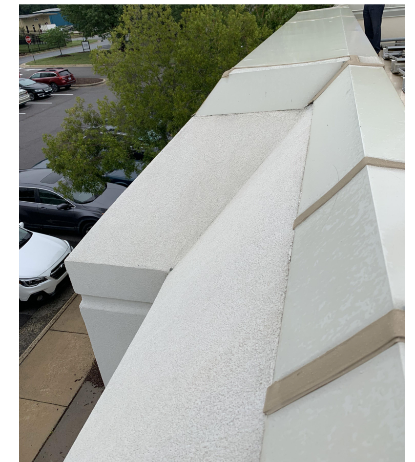
VIEW OF EAST ROOF ELEVATION LOOKING SOUTH
