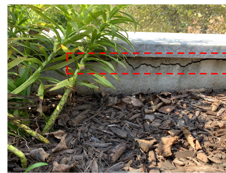
PARGE IMAGE 5 - PARGE COAT REPAIR WITHIN EXISTING PLANTERS
