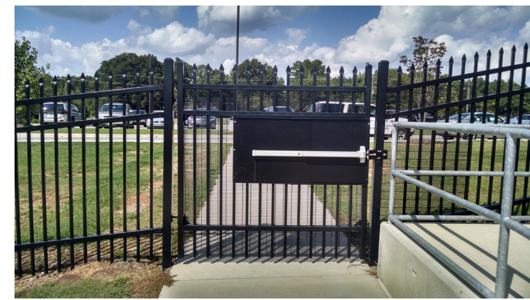
TYPICAL PEDESTRIAN GATE PANIC HARDWARE
