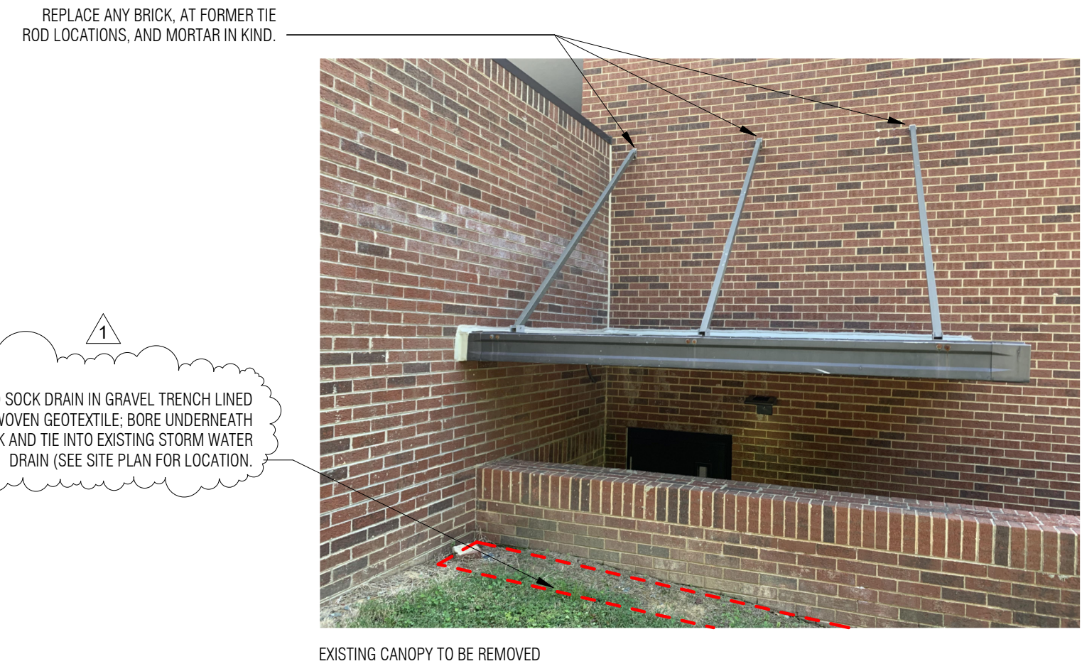
5 PARTIAL NORTH ELEVATION AT NEW CANOPY 3/16" = 1'-0"
