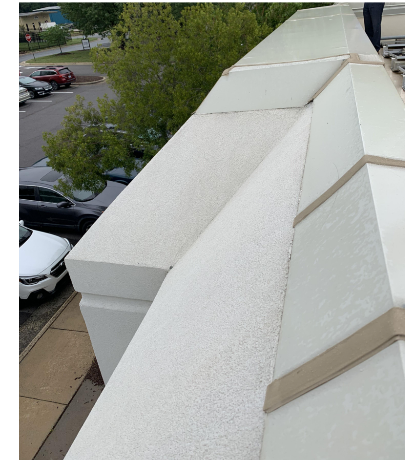
VIEW OF EAST ROOF ELEVATION LOOKING SOUTH
