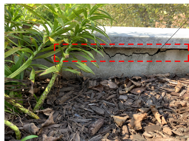
PARGE IMAGE 5 - PARGE COAT REPAIR WITHIN EXISTING PLANTERS
